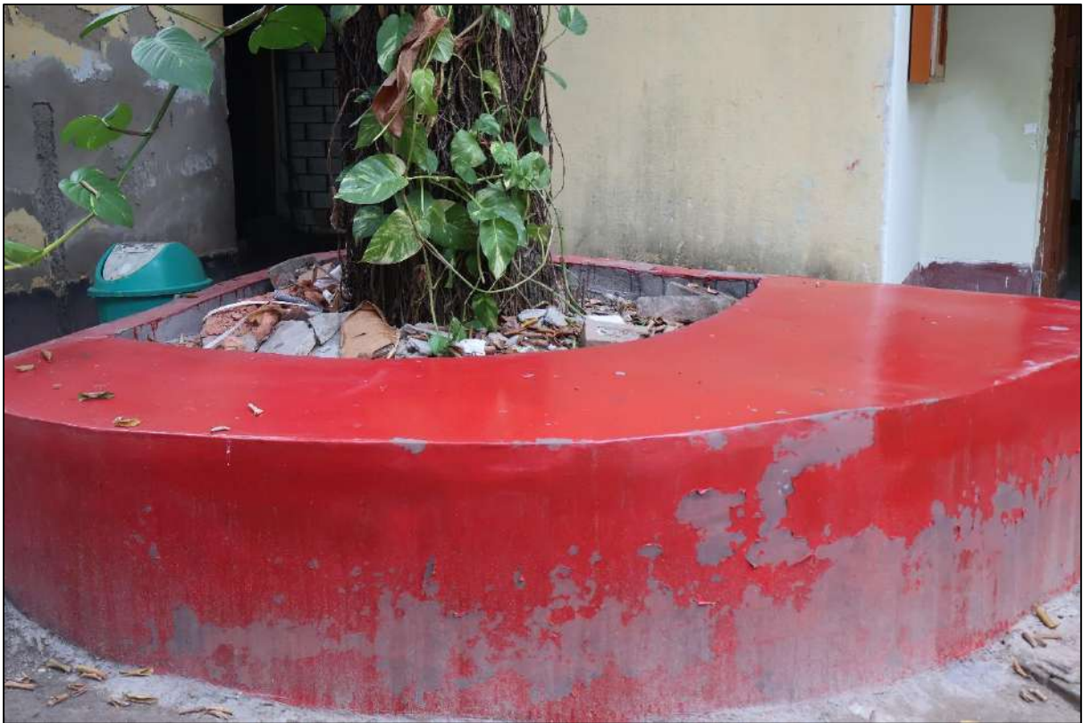
Figure 12: Concrete block around the tree
